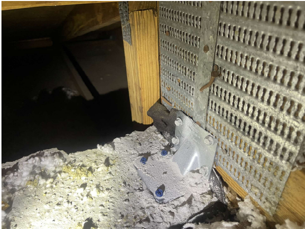
Roof to wall attachment - Clips
