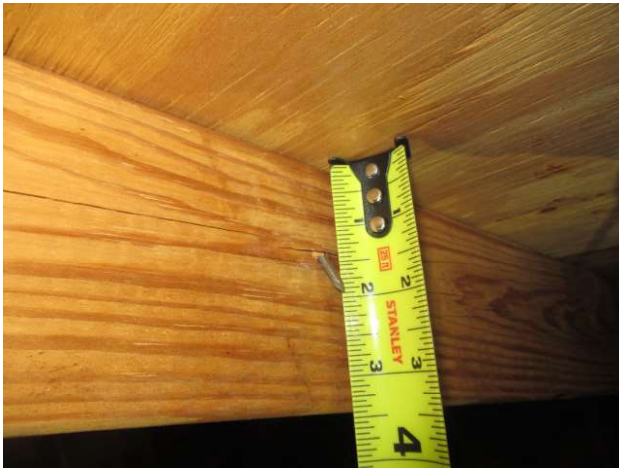
Roof deck attachment - 8d nails
