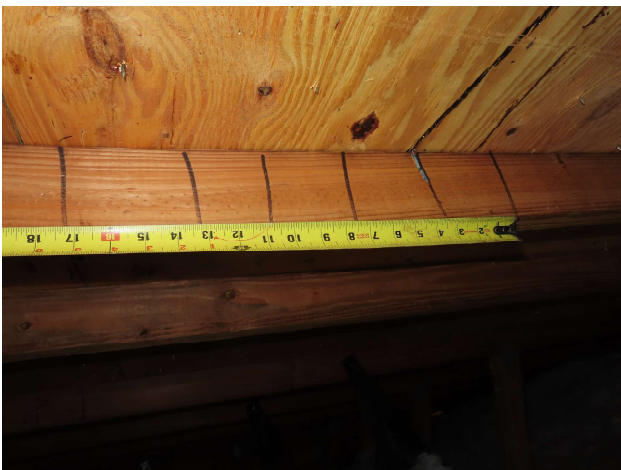
Roof deck nail spacing - Edge
