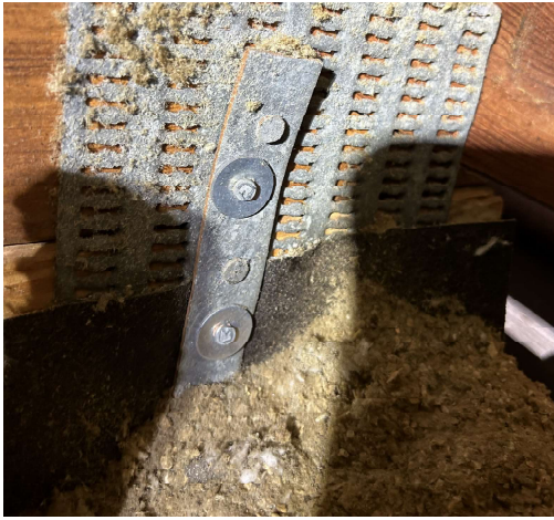
Roof to wall attachment - Clips
