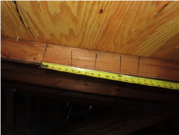
Roof deck nail spacing - Field
