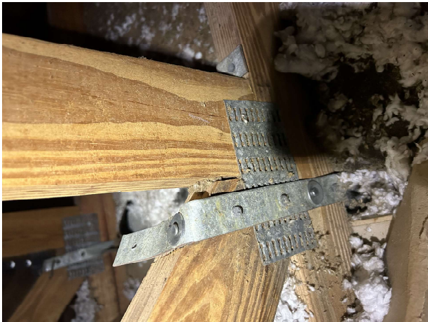
Roof to wall attachment - Clips
