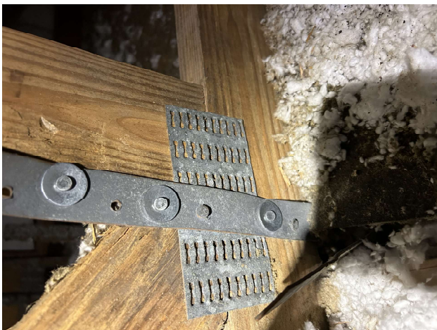
Roof to wall attachment - Clips
